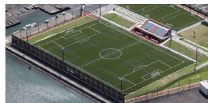
Main court with whole-surface artificial turf
